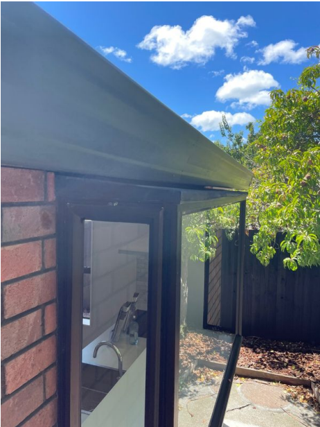
Side roof: Material Rubber Membrane
