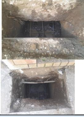
The reinforcement for the underpinning pads installed.
