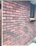
Cracks on the exterior brick veneer cladding repaired.
