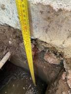
The pad excavation depth of min. 600 mm below NGL verified.
