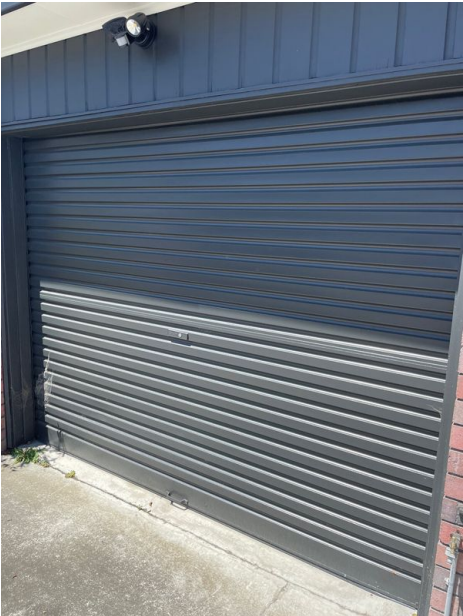
Garage Door: Material & Type Metal, Automatic, Roll-Up
