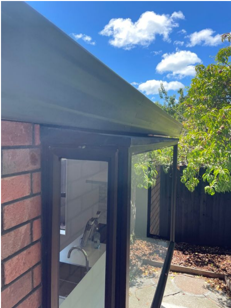
Side roof: Material Rubber Membrane
