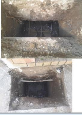
The reinforcement for the underpinning pads installed.
